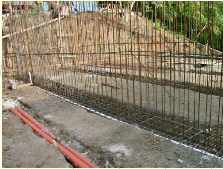
These vertical steels will eventually be encased in concrete and will become water tank walls
