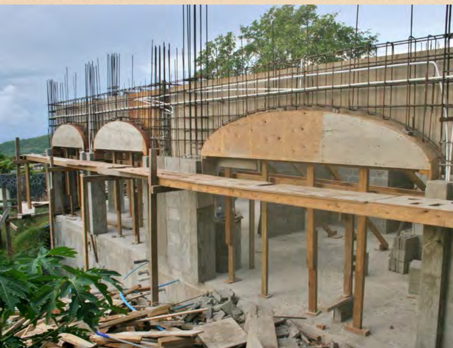
Above. Shows the Ocean View bedroom together with the laundry room and the curved wall where a spiral staircase will eventually connect up to the kitchen level. Other photos clockwise, pouring the concrete for the Ocean View bedroom floor, removing the plywood casings from the columns, building the internal walls, putting the pipework into the ring beam and preparing the arches before pouring the concrete.
