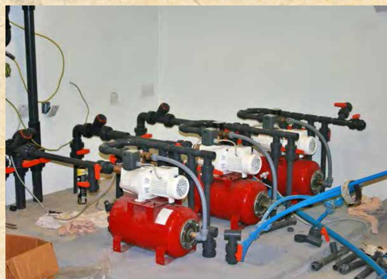
Above. Three pumps for the drinking water, pool and gardens. Pipes buried in concrete Left. The sand filter and heat exchanger used for filtering and heating the pool.
