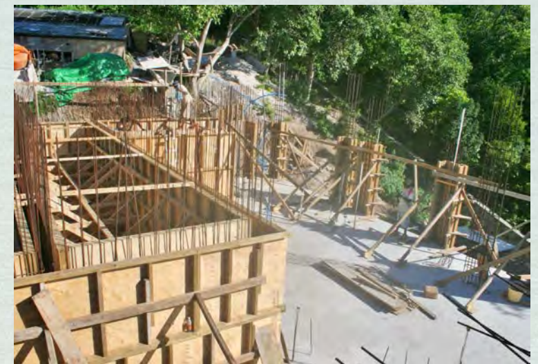
Months of work went into the formwork which eventually would be filled with concrete. Everything is supported and braced as the forces can be huge when you pour concrete.
