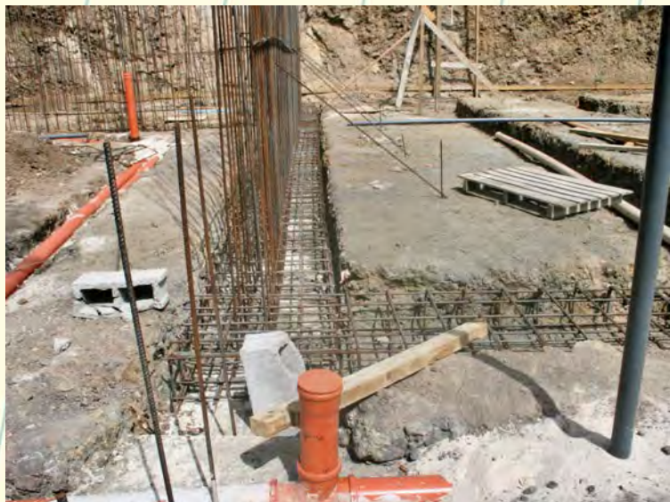
Every pipe was precisely positioned. The larger pipes were laid under the concrete floors to avoid any structural weakness.
