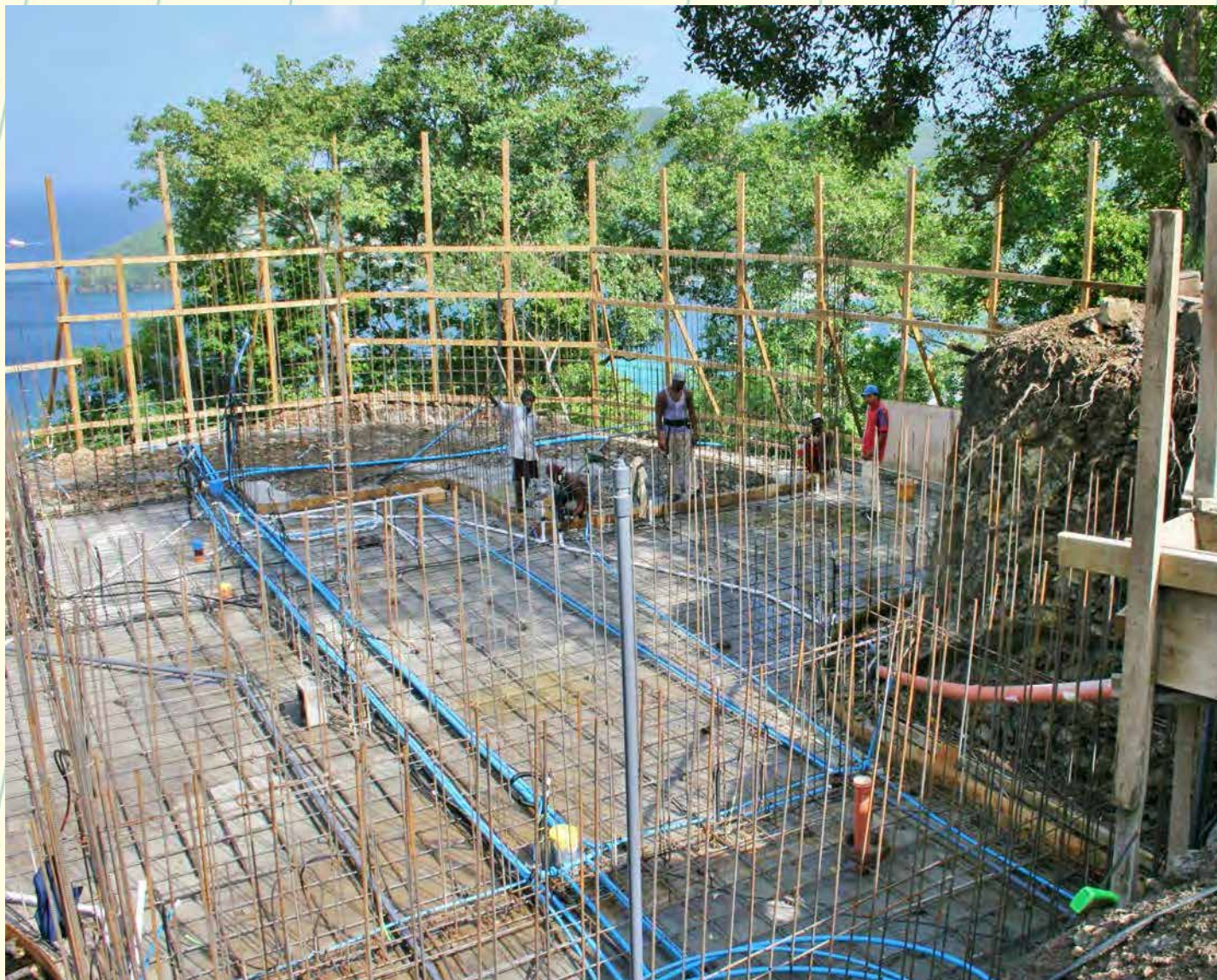
Above. Me, Julie, Samantha and Dean laying the pipes to be cast into the concrete floor.
