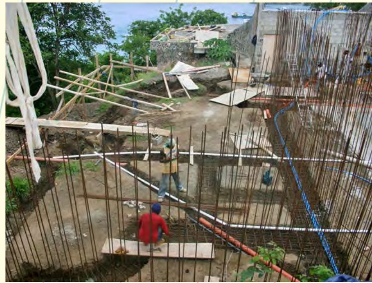
These vertical steels will eventually be encased in concrete and will become water tank walls
