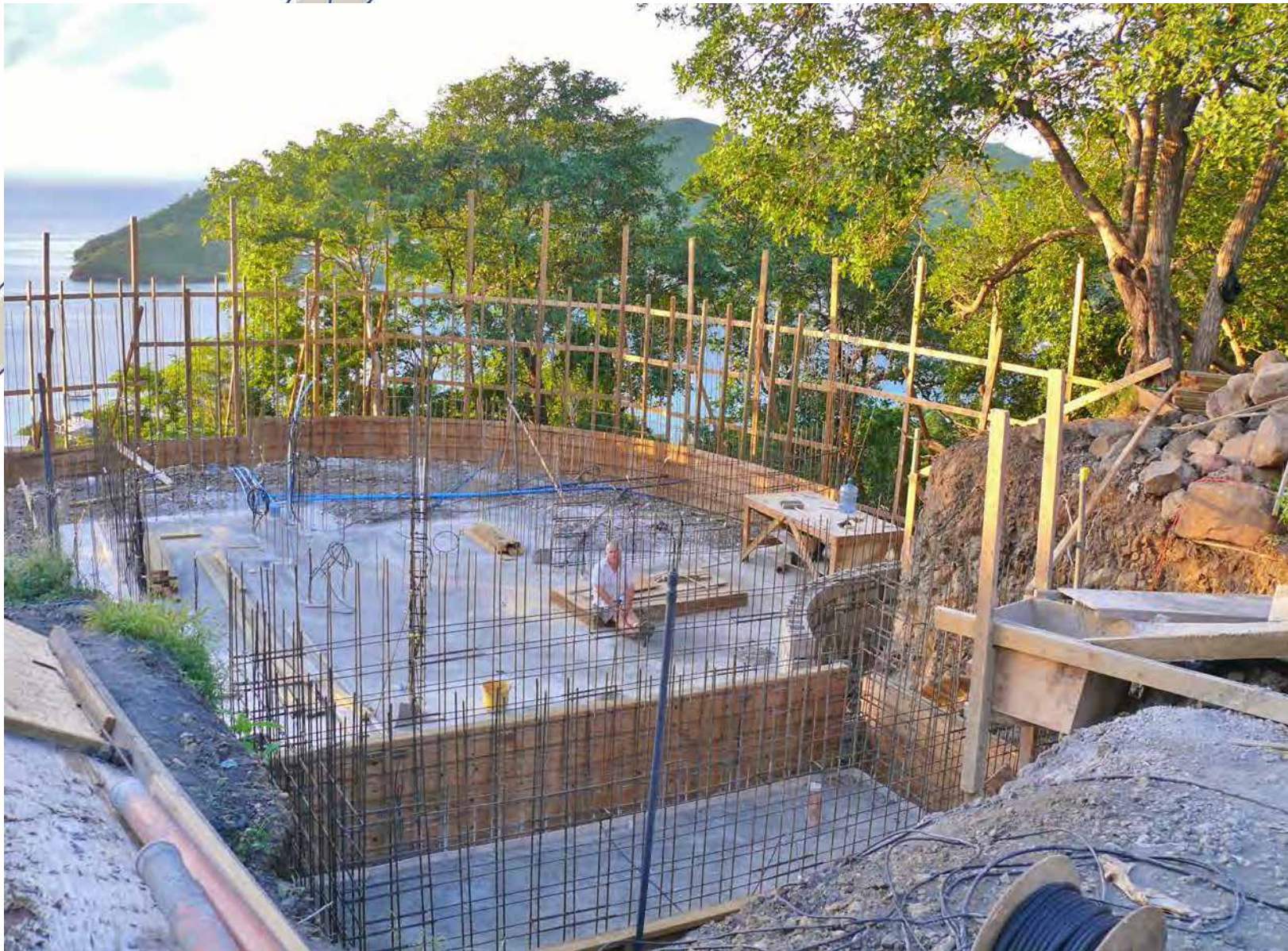
Below. Infinity Pool footings with structural vertical steels cast into the concrete.
