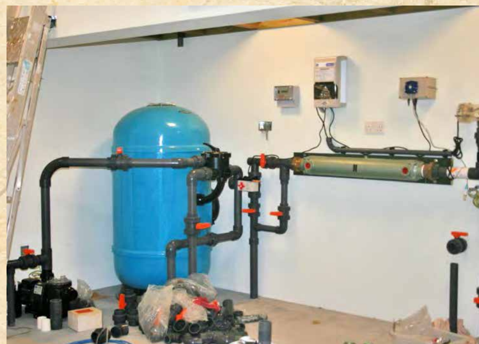
Above. Three pumps for the drinking water, pool and gardens. Pipes buried in concrete Left. The sand filter and heat exchanger used for filtering and heating the pool.
