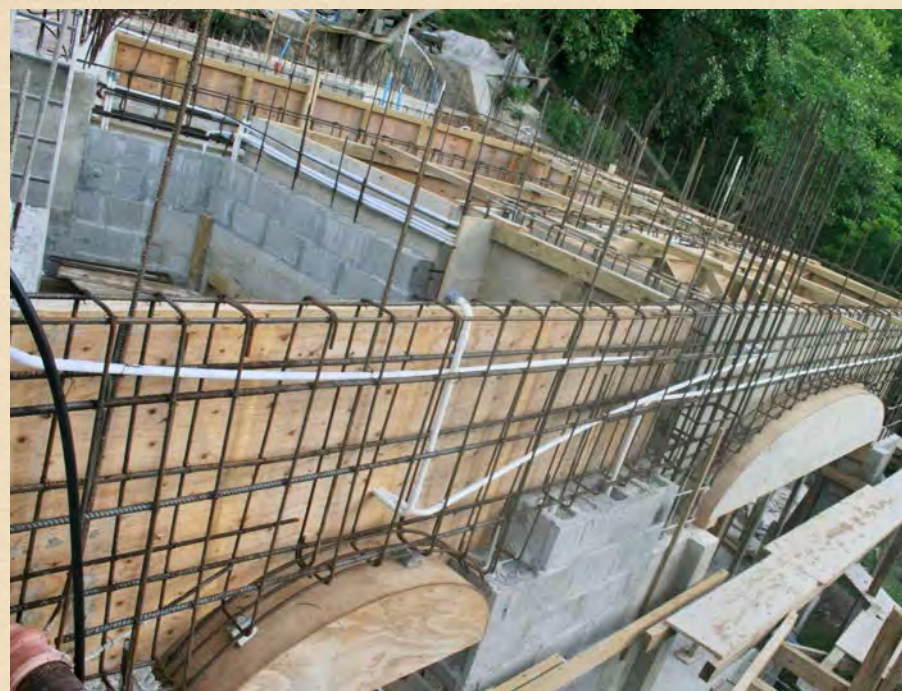
Above. Shows the Ocean View bedroom together with the laundry room and the curved wall where a spiral staircase will eventually connect up to the kitchen level. Other photos clockwise, pouring the concrete for the Ocean View bedroom floor, removing the plywood casings from the columns, building the internal walls, putting the pipework into the ring beam and preparing the arches before pouring the concrete.
