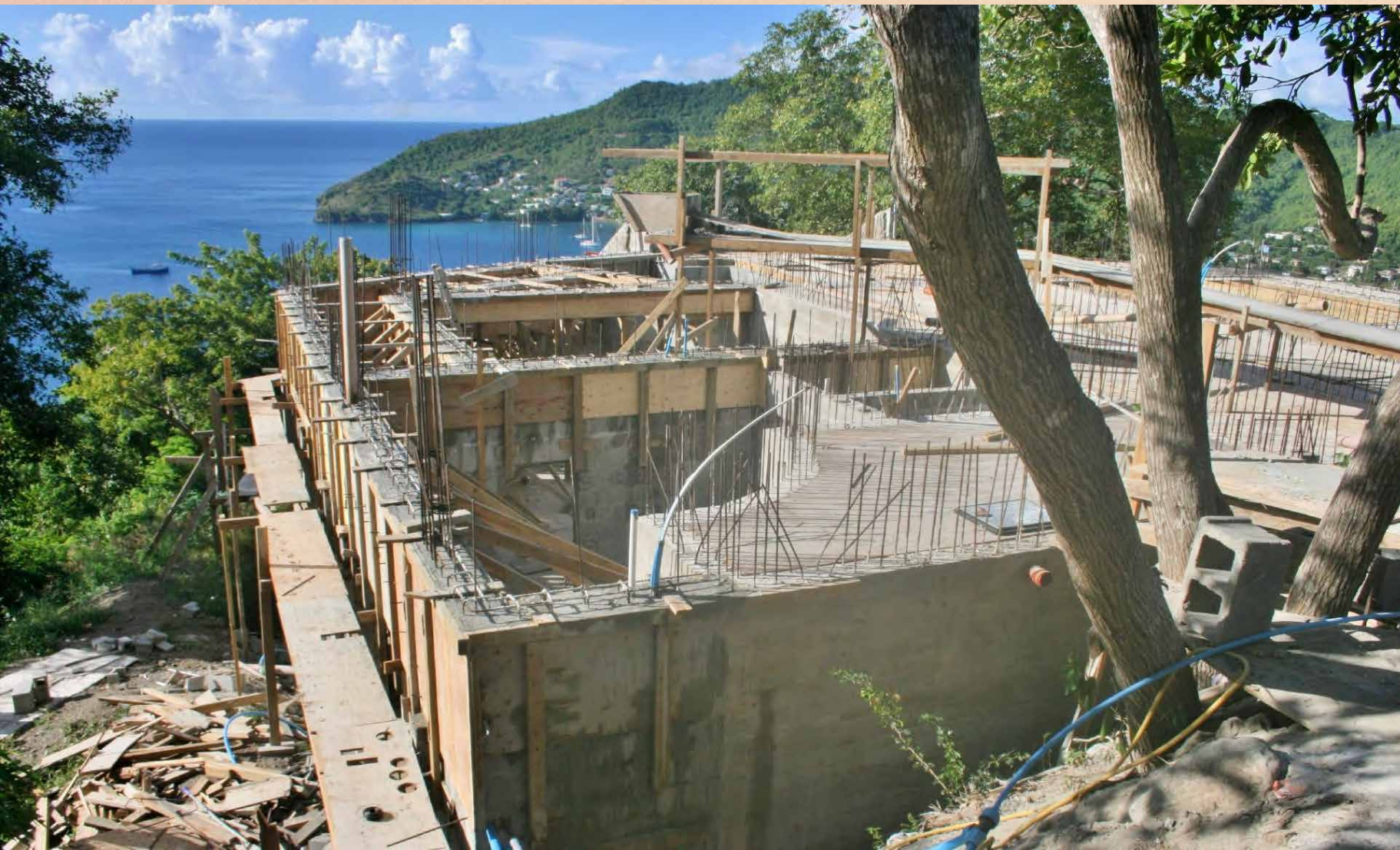
Above. Shows the Ocean View bedroom together with the laundry room and the curved wall where a spiral staircase will eventually connect up to the kitchen level. Other photos clockwise, pouring the concrete for the Ocean View bedroom floor, removing the plywood casings from the columns, building the internal walls, putting the pipework into the ring beam and preparing the arches before pouring the concrete.
