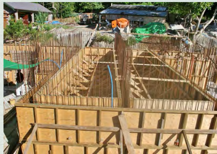
Months of work went into the formwork which eventually would be filled with concrete. Everything is supported and braced as the forces can be huge when you pour concrete.
