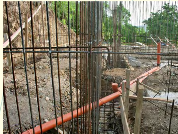
Every pipe was precisely positioned. The larger pipes were laid under the concrete floors to avoid any structural weakness.
