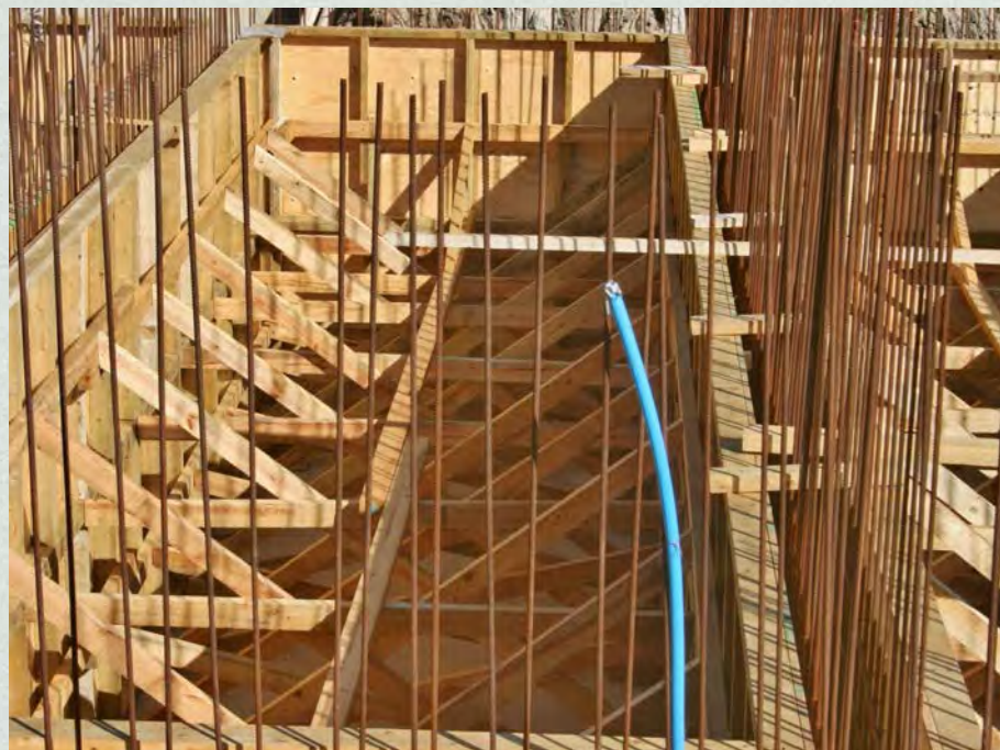
Months of work went into the formwork which eventually would be filled with concrete. Everything is supported and braced as the forces can be huge when you pour concrete.
