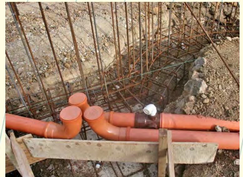
Every pipe was precisely positioned. The larger pipes were laid under the concrete floors to avoid any structural weakness.
